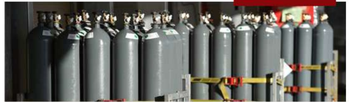
Storage Tanks and Cylinders (Flammable & Combustible)
